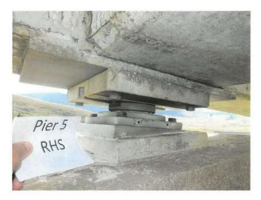
Figure 8 Example of guided bearing with tapered bottom plate
