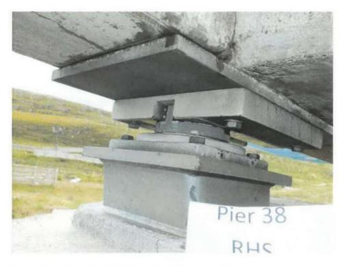
Figure 10 Example of guided bearing with bottom steel shoe
