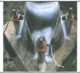
Photographic record showing Anchor Bolts/Washers and Cone to Tower Weld on Tower 9. High tensile wires are termination points for snow fences following the tow up the hill.
