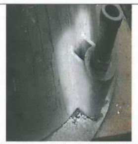
Photographic record of Base Plate and Anchor Bolt Housing on Tower 3. Restrictions encountered on internal Anchor Bolt Housing.
