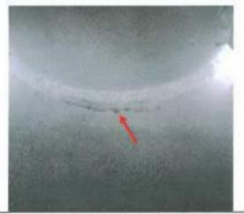
Photographic record showing undercut on Tower to Deck Connection weld on Tower E down-hill facing.
