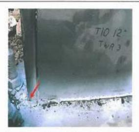
Photographic record showing 4mm indication on Stiffener to Deck Connection weld on Tower 3 Up-hill right hand side.
