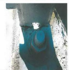
Photographic record showing base plate connection welds from angled lattice work and anchor bolt on T1L (facing down-hill).
