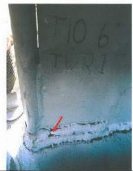
Photographic record showing 20mm indication on downward Left hand Stiffener web on Tower 1.
