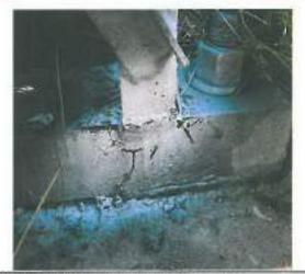
Photographic record showing Base Plate connection weld from lattice tower facing down-hill on T3L.
