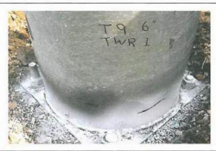
Photographic record of Base Plate Connection weld to Tower 1 looking down-hill (6 o'clock). No restrictions were encountered and no indications found.
