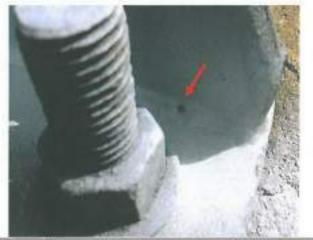
Photographic record showing Porosity on Stiffener Deck Connection weld on Right hand side down-hill Stiffener on Tower E.
