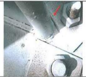
Further Photographic record showing Anchor Bolts and Washers restricting inspection of Weld Cap and HAZ on Tower 6.
