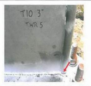
Photographic record showing 25mm indication on Web Stiffener Trim on Tower 5 at 3 o'clock Position (looking up hill). Indication does not affect structural integrity of Stiffening Web.
