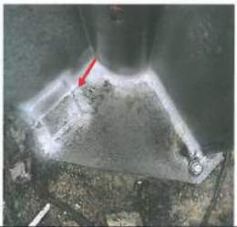
Photographic record showing Extra "L-Plate" weldment to Stiffener web on Tower 7. No Restrictions were encountered and No Indications found.
