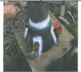
Photographic record showing extent of Magnetic Particle Inspection area at Base Plate Cone to Tower and Housing Welds and Anchor Bolts on Tower 6.
