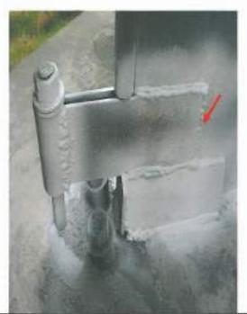
Photographic record of Base Plate Connection weld to Stiffener web configuration on Tower 2. Porosity Found throughout Anchor Bolt Housing to Web welds.
