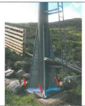
Stand-off Photographic record of Base Plate and Stiffeners on Tower 2. Red Arrows indicate Anchor Bolts and washers impeding inspection of Stiffener Foot Weld and HAZ.
