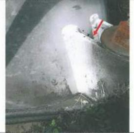
Photographic record showing Anchor Bolt Housing and internal Restricted Inspection area on Tower 6.
