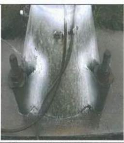
Photographic record of Base Plate Cone and Anchor Bolts and Housings on Tower 7.
