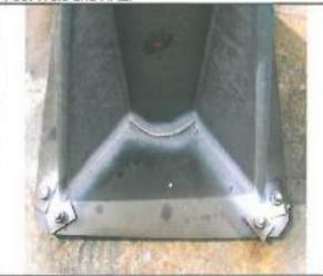
Photographic record showing 25% of inspection area of Base Plate Welds and Anchor Bolts and Washers on Tower 6.
