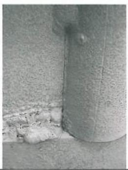
Photographic record showing 55mm indication on Base Plate Stiffener Web Trim (Non Structural) on T2.
