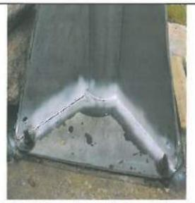
Stand-off Photographic record of Base Plate and Anchor Bolts on Tower 2. No Restrictions encountered. A 7mm Indication was found on the right hand side Stiffener facing down-hill.
