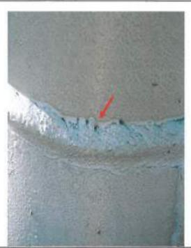
Photographic record showing Porosity on right hand side Cone to Tower Weld facing down-hill on Tower 11 indicated by red arrow.
