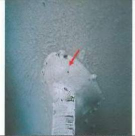
Photographic record showing Porosity at 10 o'clock Anchor Bolt Housing facing up hill on Tower 9.
