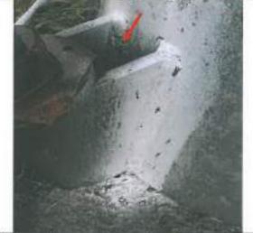
Photographic record of Base Plate Cone and Anchor Bolts and Housing on Tower 15. Arrow indicates restricted access to internal Anchor Bolt Housing.
