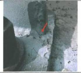
Photographic record showing 11mm Indication at foot of Stiffener web on Left hand side up-hill Stiffener on Tower 9.
