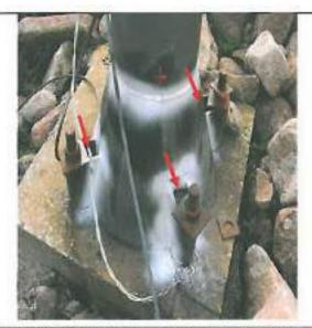
Stand-off Photographic record of Base Plate Cone and Anchor Bolt Housings on tower 2. Restrictions encountered within housings indicated by red arrows.
