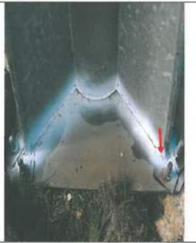
Photographic record showing Deck Plate and Stiffener welds with Anchor bolts on Tower 2.
