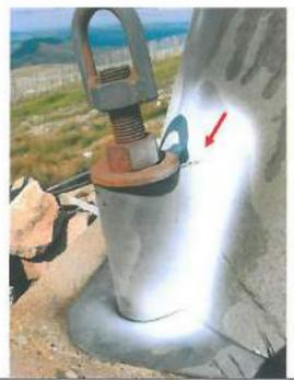
Photographic record of Base Plate and Anchor Bolt Housing on Tower 2. Restrictions were encountered on internal Base Cone Connection from Anchor Bolt Housing.
