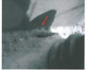
Photographic record showing Porosity on Stiffener Deck Connection weld on left hand side down-hill Stiffener on Tower 9.
