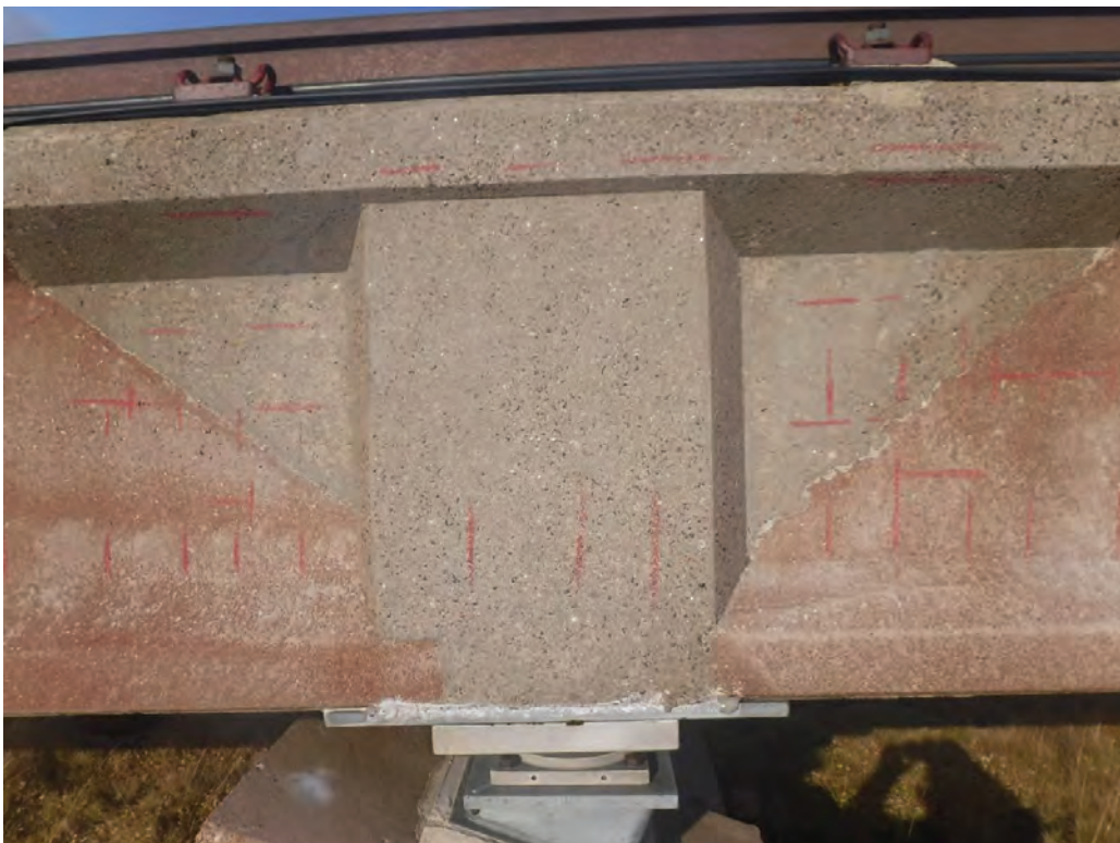
Plate 48 - General view of surface markings to Pier 80 Right Beam up/down
