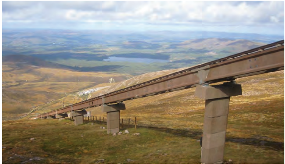
Figure 2-1 Typical view of structure
