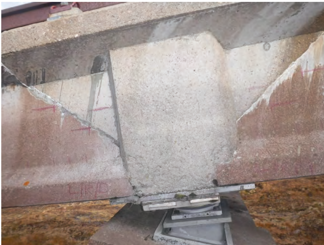
Plate 28 - General view of surface markings to Pier 54 Right Beam, left support up/down
