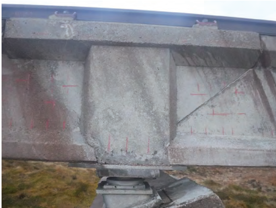
Plate 38 - General view of surface markings to Pier 69 Left Beam Up
