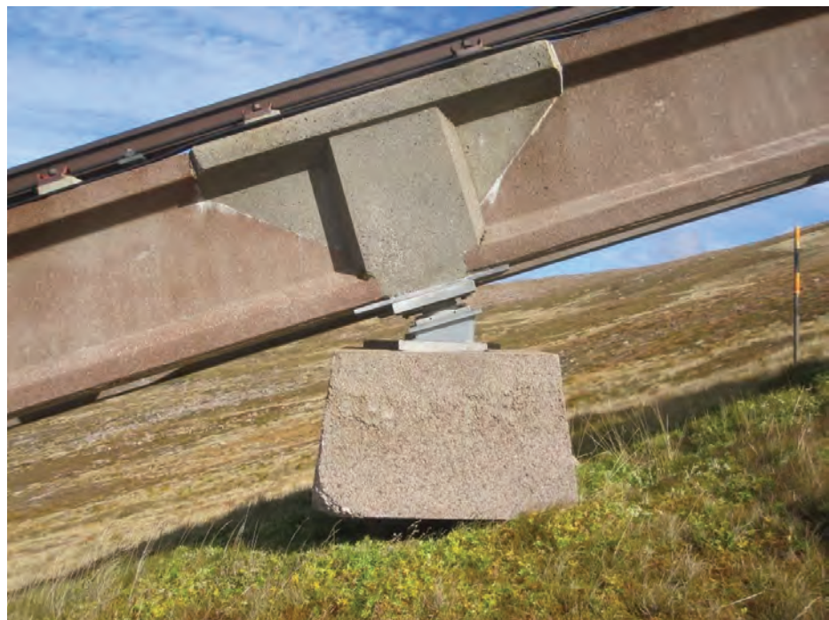
Figure 2-3 Typical insitu stitch at support
