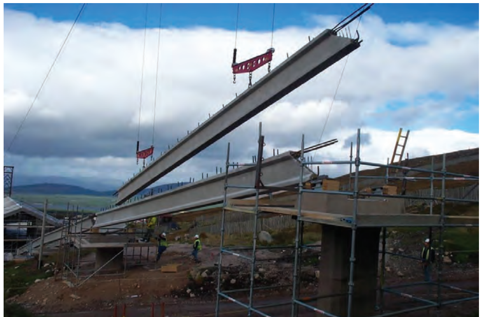
Figure 3-1 Precast beam installation
