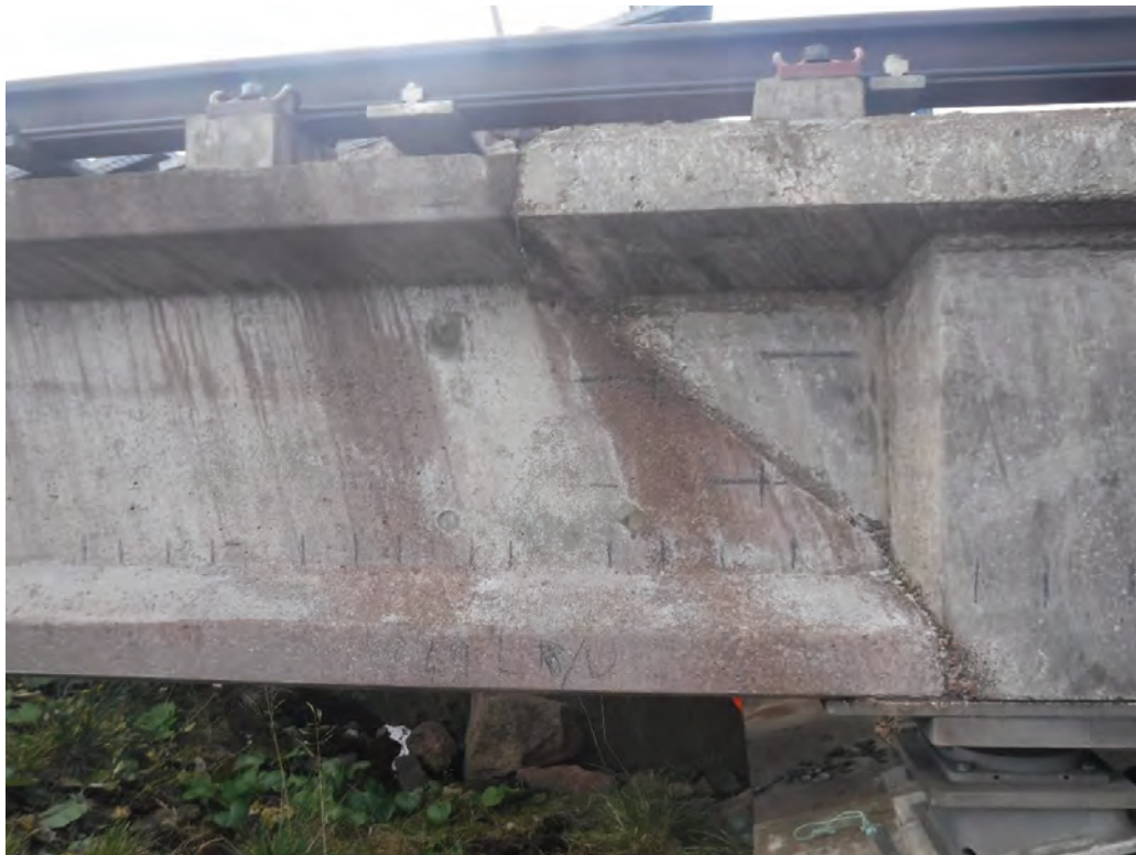
Plate 14 – General view of surface markings to Pier 49 Left Beam up
