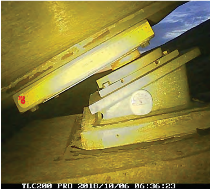
Figure 9 - Pier 91, extremity of movement
