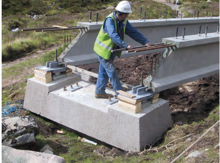
Figure 4-2 Beam end details
