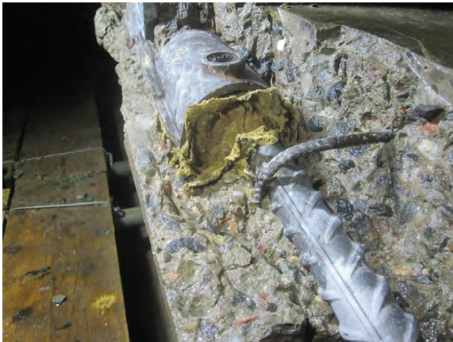
Figure 9 DENSO tape at grouted coupler end
