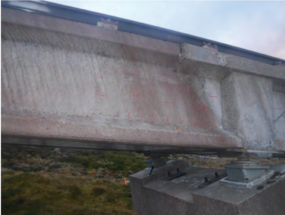
Plate 37 - General view of surface markings to Pier 69 Left Beam Up
