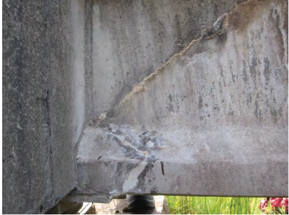
Figure 2-7 Crack repair at pier 9 (refer defect 1)
