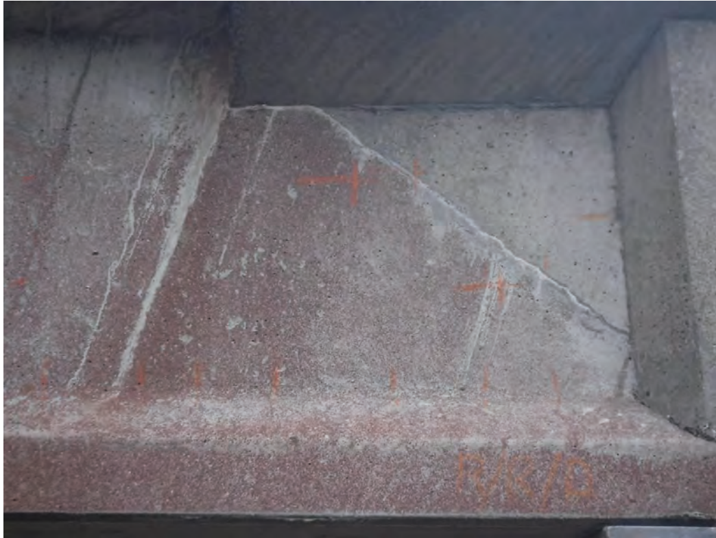
Plate 25 - General view of surface markings to Pier 53 Right Beam, right support down.
