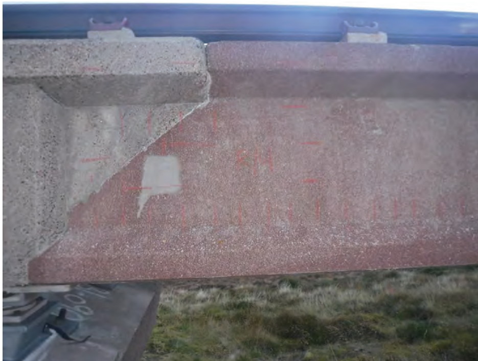
Plate 34 - General view of surface markings to Pier 69 Right Beam up
