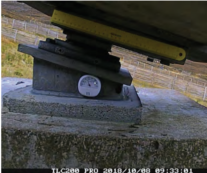
Figure 3 - Pier 44, extremity of movement
