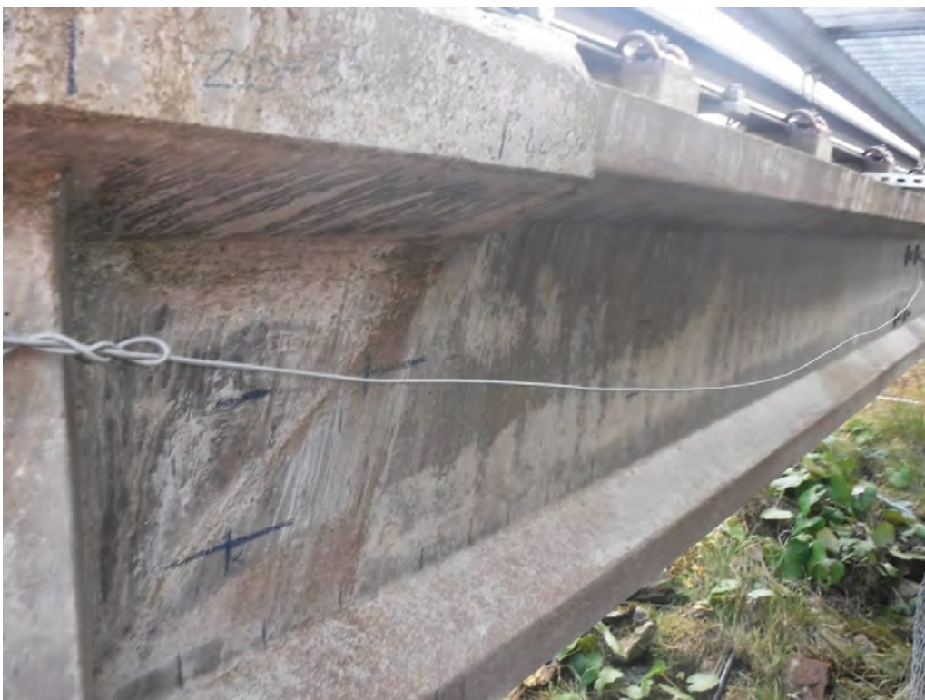
Plate 16 – General view of surface markings to Pier 49 Right Beam up
