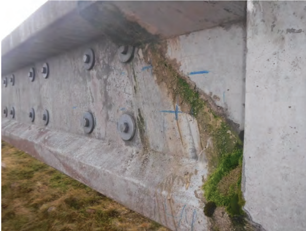
Plate 33 - General view of surface markings to Pier 56 Left Beam up
