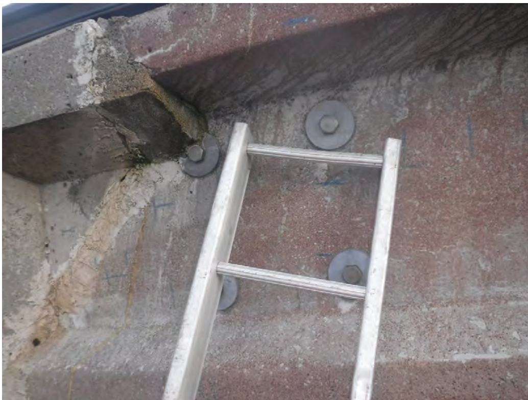
Plate 30 - General view of surface markings to Pier 56 Right Beam up
