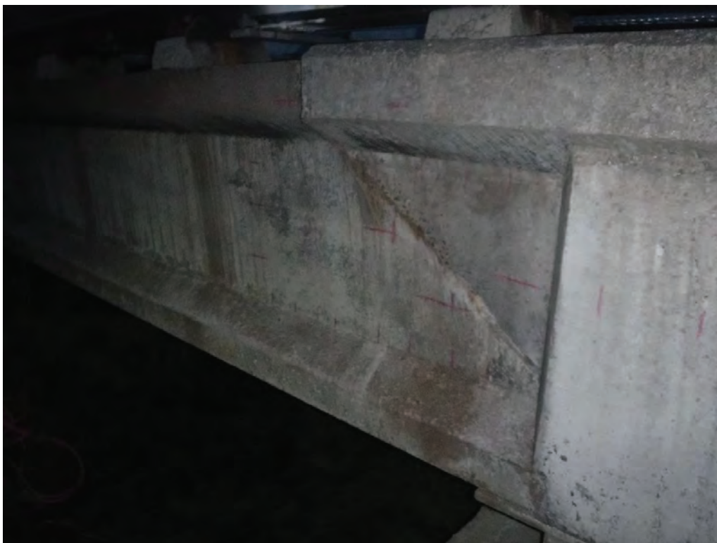
Plate 12 – General view of surface markings to Pier 22 Left Beam up
