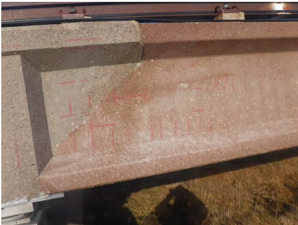
Plate 46 - General view of surface markings to Pier 80 Right Beam up
