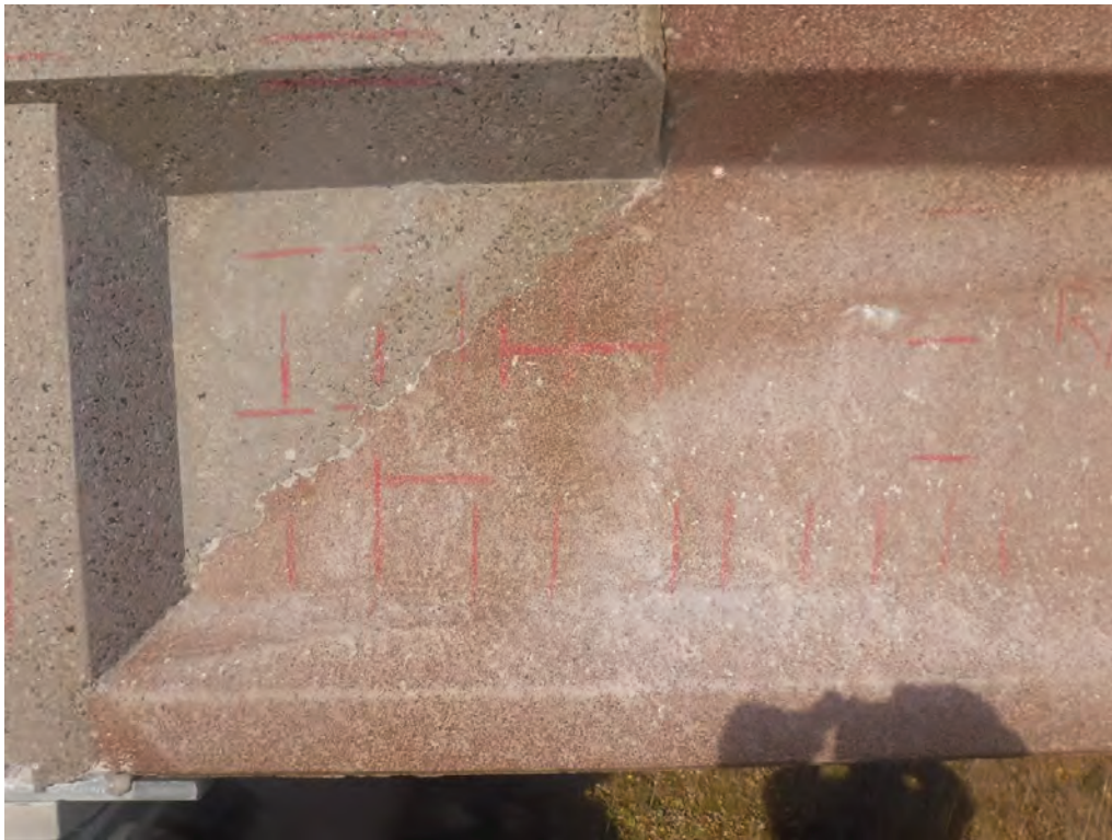
Plate 47 - General view of surface markings to Pier 80 Right Beam up
