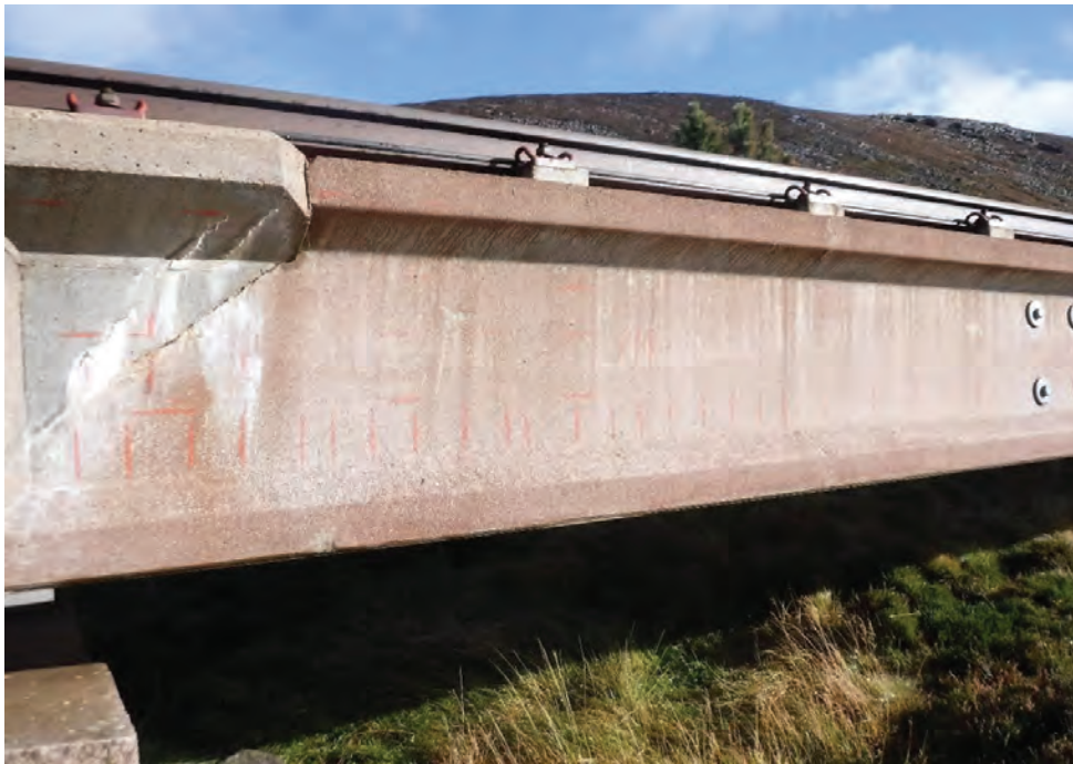
Plate 7 – General view of surface markings to Pier 9 Right Beam up
