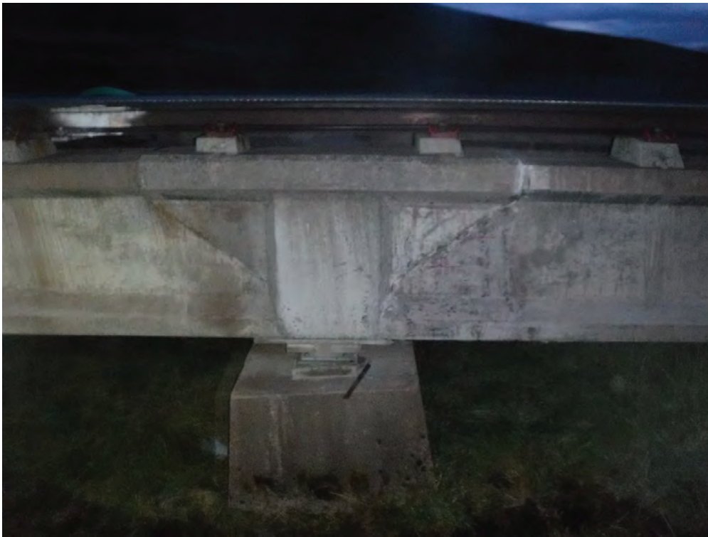
Plate 11 – General view of surface markings to Pier 22 Left Beam up/down
