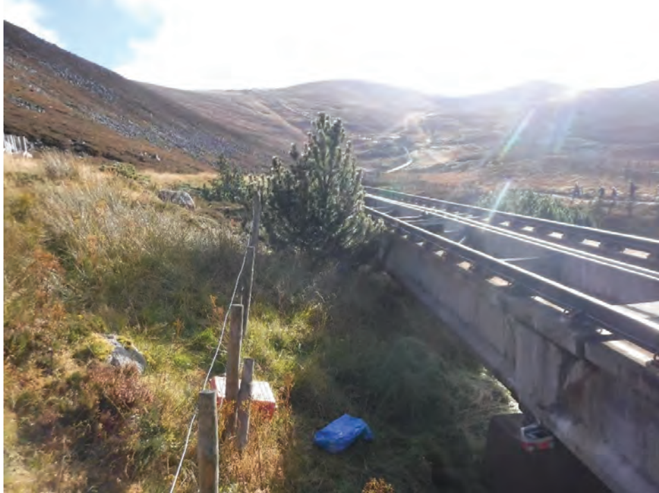
Plate 1 – General view of funicular railway.
