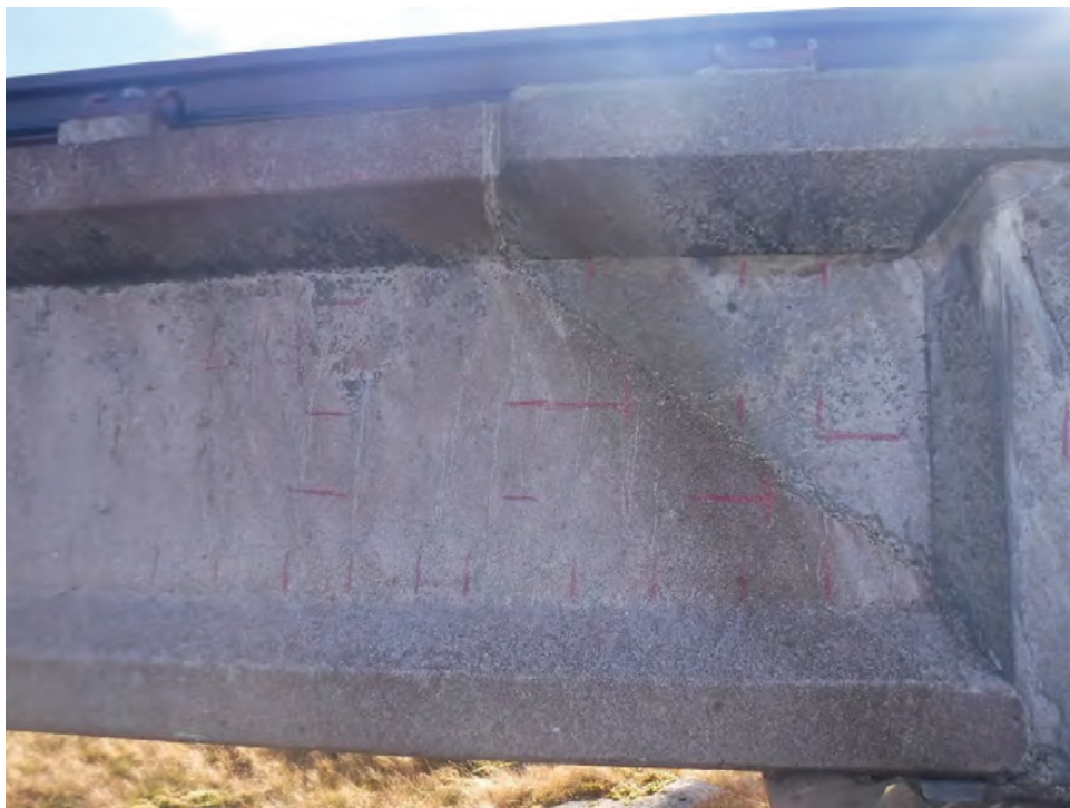
Plate 42 - General view of surface markings to Pier 80 Left Beam up
