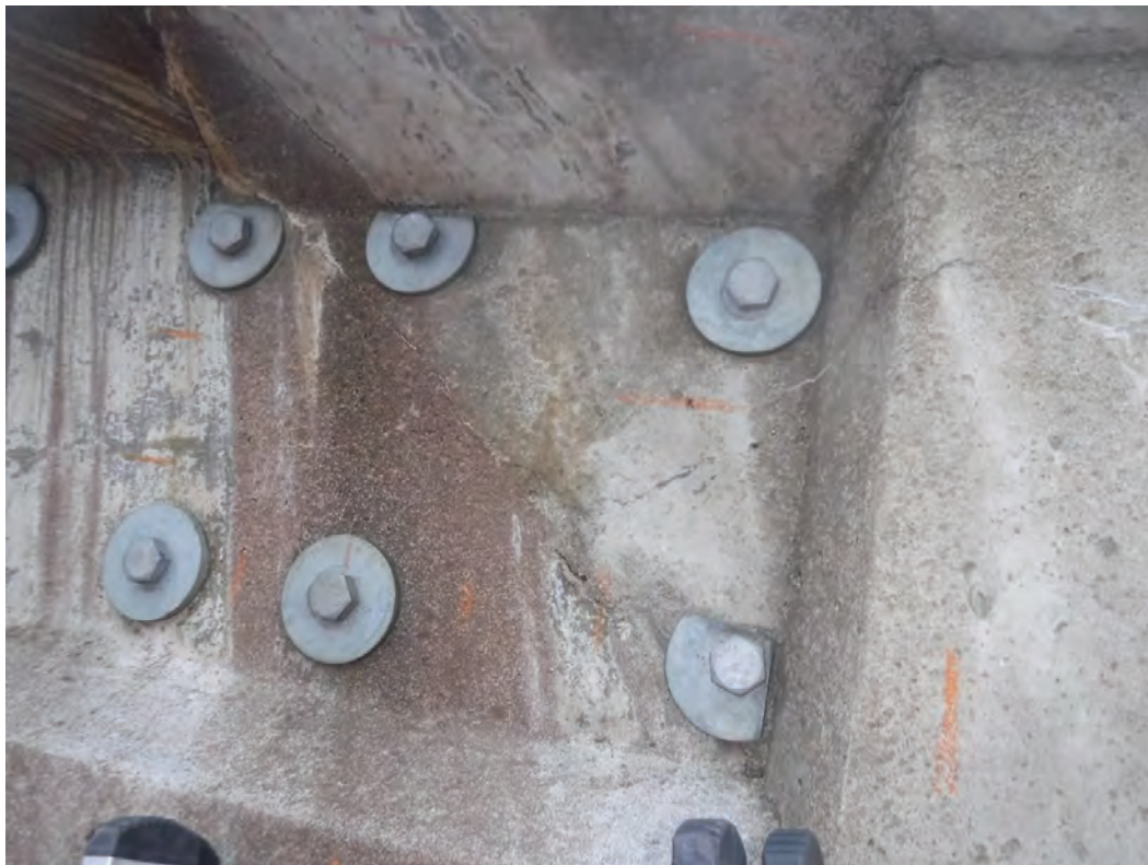
Plate 18 – General view of surface markings to Pier 51 Left Beam up
