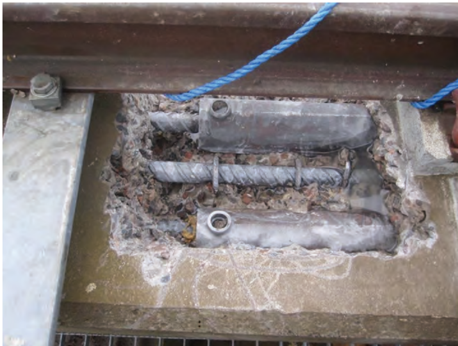
Figure 7 Breakout at pier 56 showing staggered coupler arrangement
