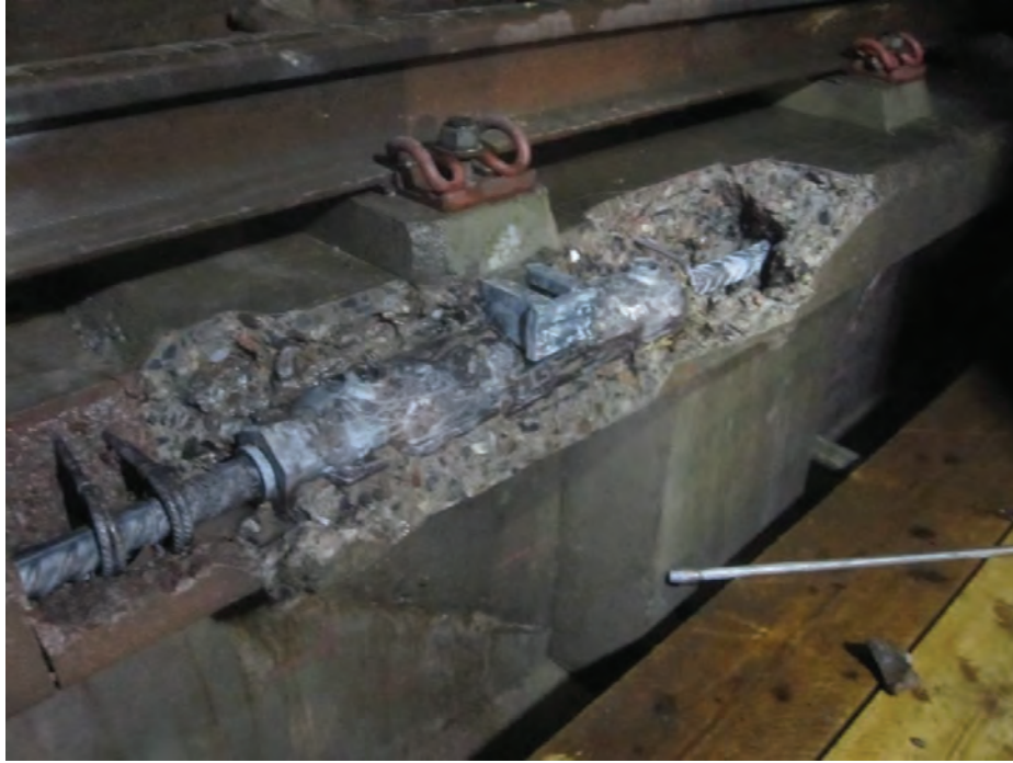
Figure 5 Exposed grouted coupler at pier 22
