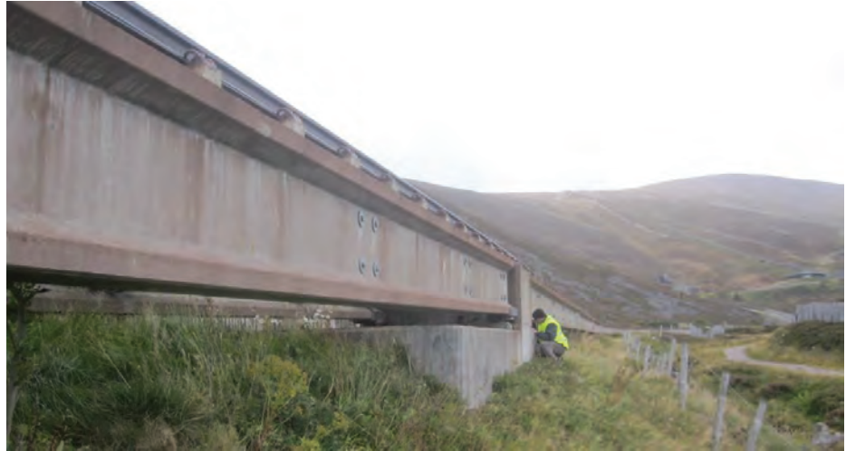
Figure 2-4 Typical anchor block
