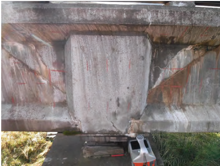
Plate 3 – General view of surface markings to Pier 9 Left beam connection.
