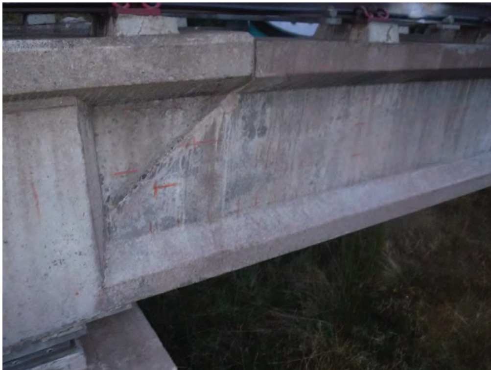
Plate 10 – General view of surface markings to Pier 22 Right Beam up
