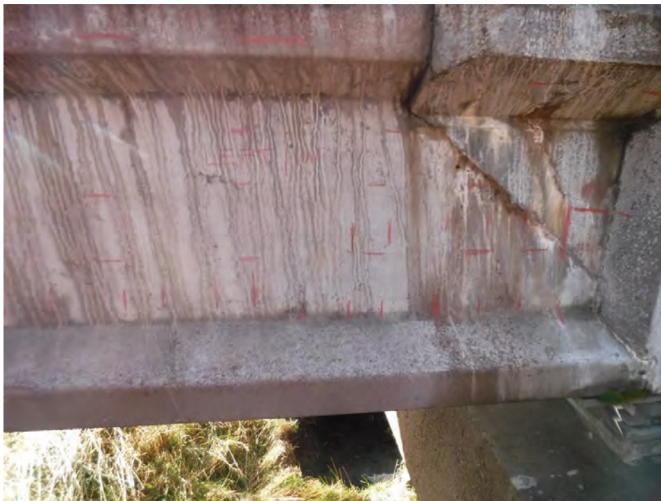
Plate 4 – General view of surface markings to Pier 9 Left Beam up.
