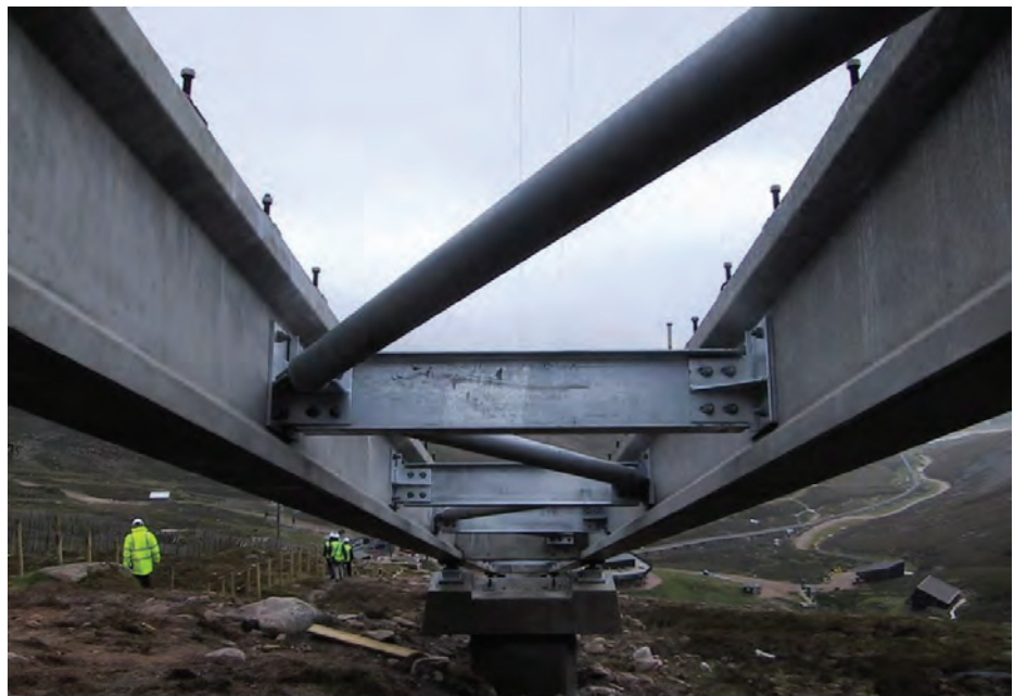
Figure 2-5 Construction photograph showing bracing
