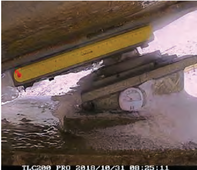
Figure 6 - Pier 61, extremity of movement
