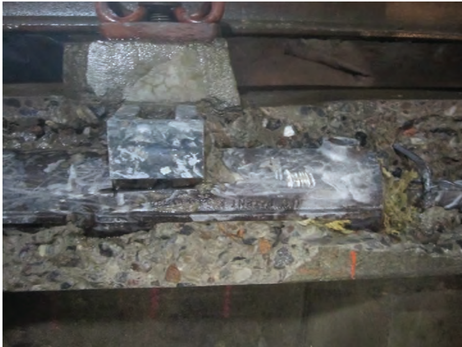
Figure 6 Close-up view of grouted coupler cut-out around HALFEN channel at pier 22
