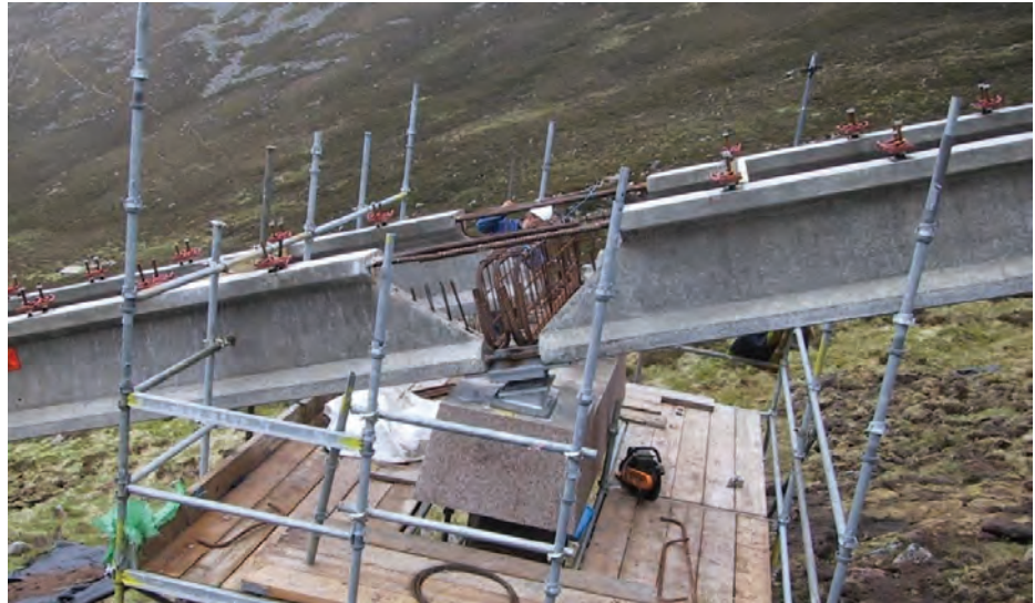
Figure 3-2 Construction of insitu splice
